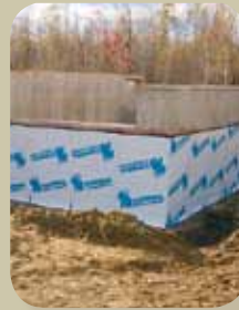
COLPHENE 3000 Self-adhesive membrane for foundation waterproofing
