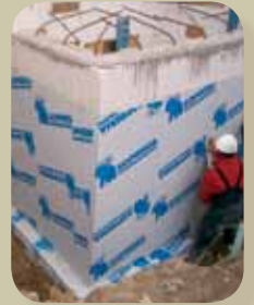
COLPHENE ICF Self-adhesive membrane for insulated concrete form waterproofing
