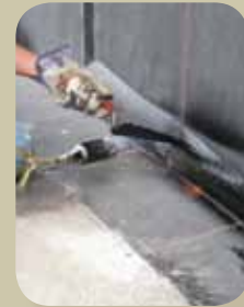
COLPHENE TORCH N' STICK SBS modified bituminous membrane uses on foundations walls and other vertical below grade concrete surfaces
