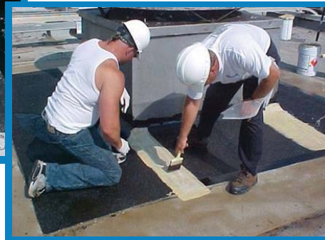
3. Repair with: Alsan Trafik HP 520 and Reinforcement
