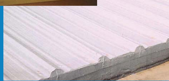
Metal Roof After
