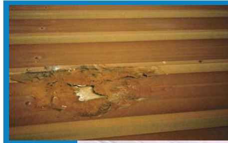
Metal Roof Before
