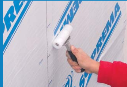
Fully adhere membrane using a hard roller.
