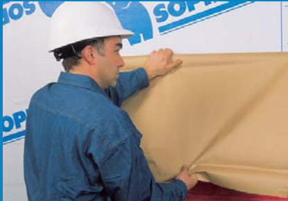
Making sure the alignment is correct, remove the silicone release paper completely.
