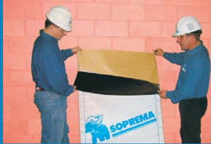
Remove the top portion of the silicone release paper.
