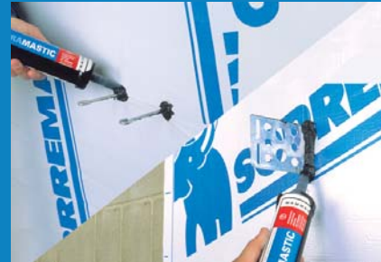
Use a Sopramastic to seal around penetrations and details.
